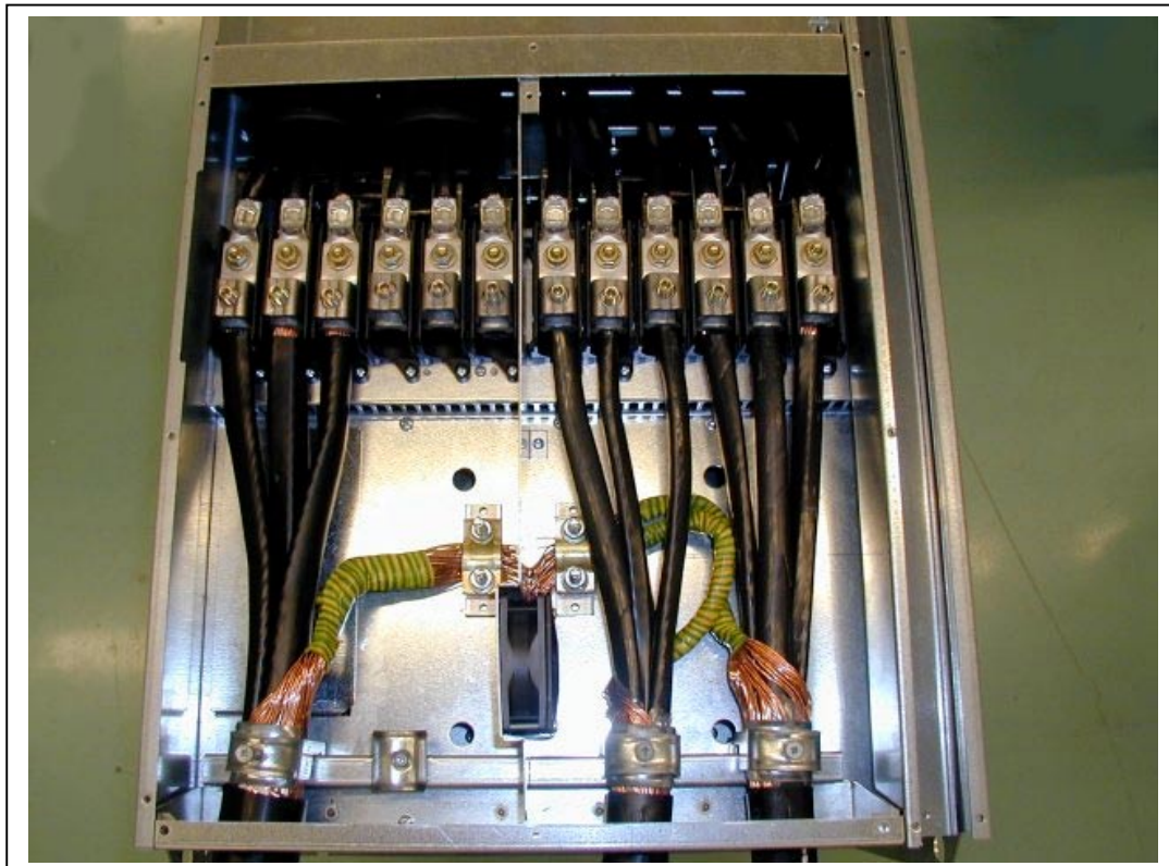
Figure 6-16. Cable installation in NX, FR9
