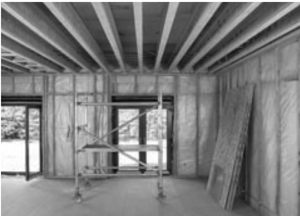
Fig. 2: Underside of joist space construction
